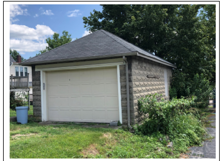
This historic garage is an important part of the streetscape of East Walnut Street. Matching ornamental concrete block was used for the foundation and porch of the house it serves.
