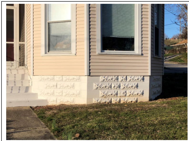
The pattern of plain and rock-faced concrete blocks on the foundation of this East Walnut Street home is an important part of its architectural character.
